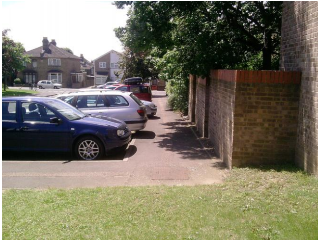
Benjamin Close looking towards Globe Road – parked vehicles overhanging footway
